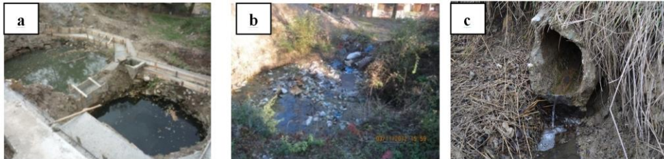
Fig. 5. The old wells and tank (a, b) and drainage channel (c) nowadays (Pictures: Meret Rodica)
