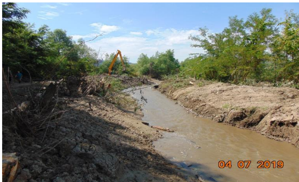
Fig. 6. Riverbed unsilt and restoring the old riverbed of Pianu river – photo C.A. SAFTA
