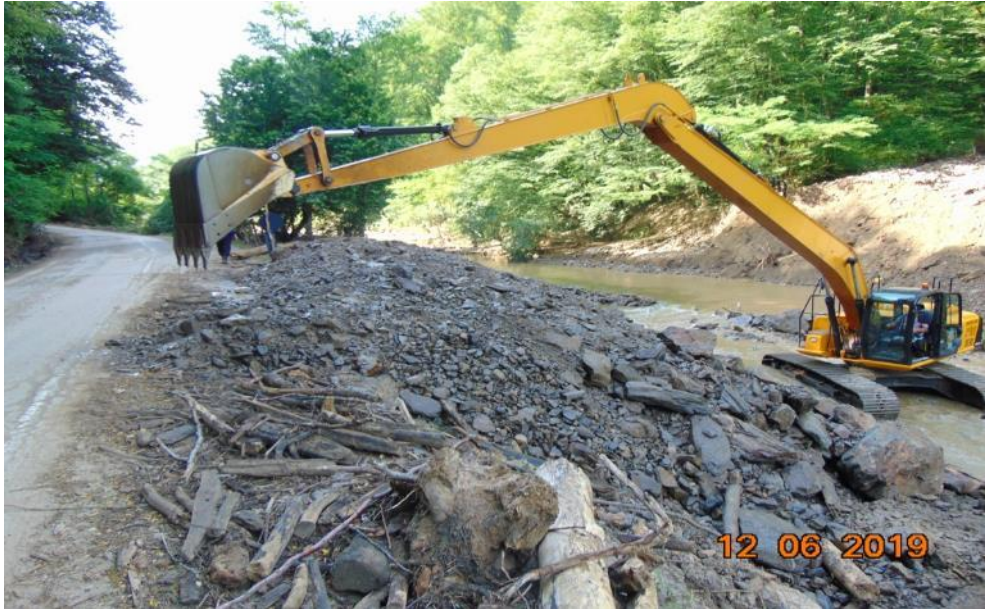
Fig. 4 Pianu riverbed recalibration – downstream of Strungari village – photo C.A. SAFTA
