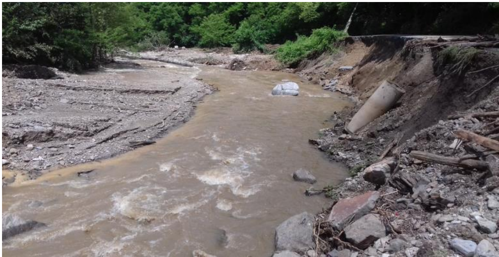
Fig. 3. Riverbed and communal road erosion – downstream of Strungari village – photo C.A. SAFTA
